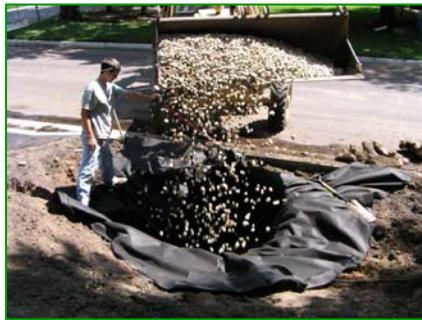
rock infiltration sump under the garden. This "rock baggie" helps water infiltrate quickly.
